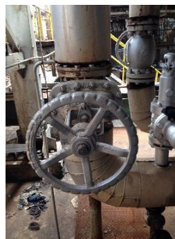
Gambar 3.4 Valve Steam exhaust
