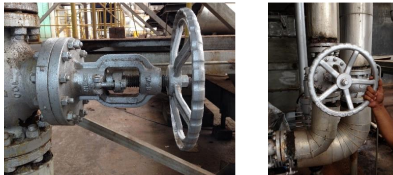
Gambar 3.3 Valve Steam Inlet
