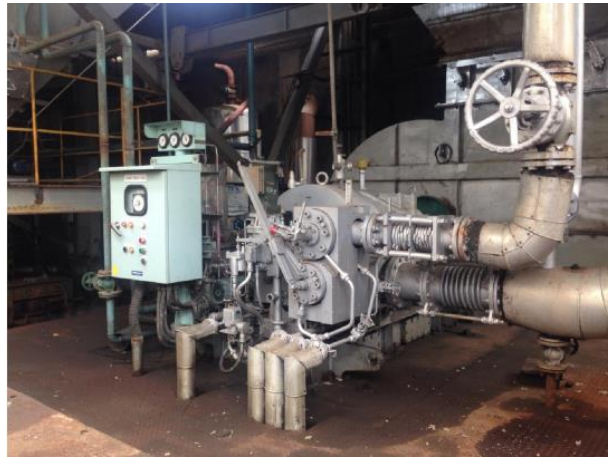
Gambar 3.1 Steam Turbine FDF
