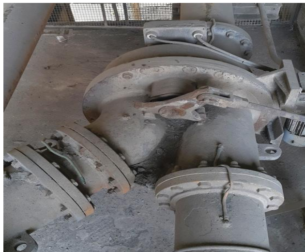
Gambar 1. Diverter gate
